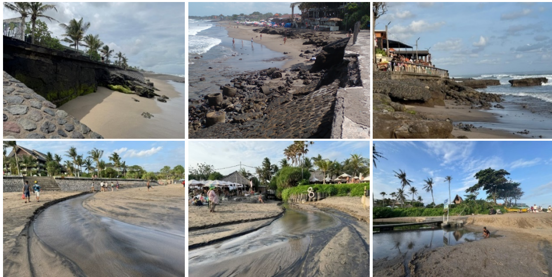
Figure 11. Seawall damage and changes in estuary flow direction
