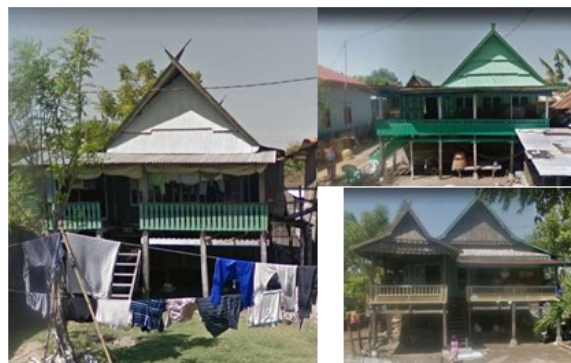
Figure 4. A view of the traditional building from the local community of Cikoang Village Source: Google Earth, 2019
